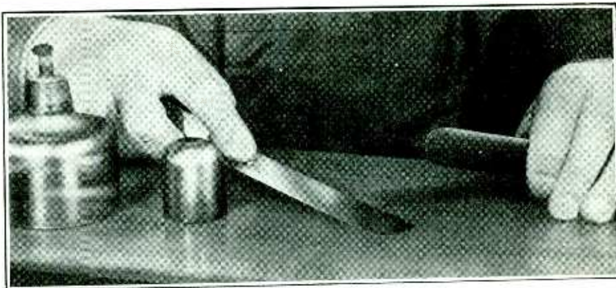
Removing dents and scratches from highly polished cabinets with a "shellac stick" by the aid of a spatula and an alcohol lamp
